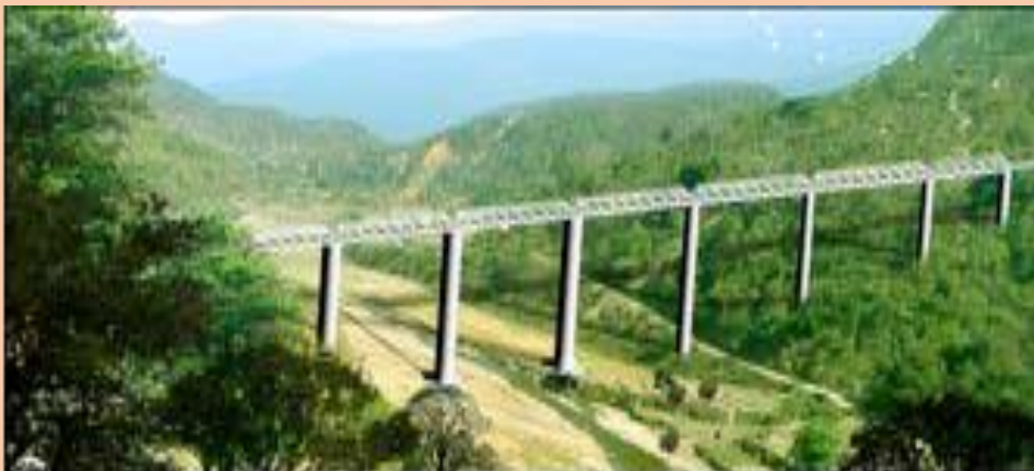
HIGHEST RAIL BRIDGE UNDER CONSTRUCTION IN NORTH EAST
