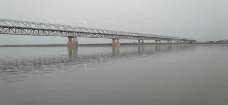
RAIL CUM ROAD BRIDGE ON GANGA - MUNGER
