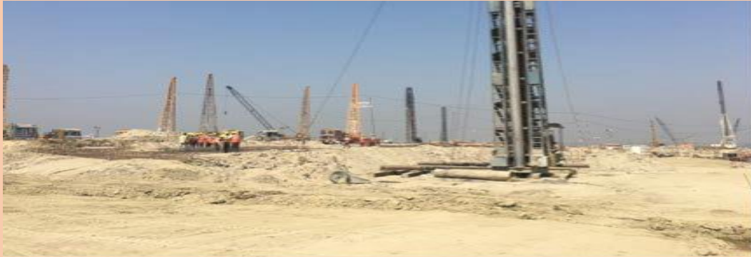
CONSTRUCTION IN FULL SWING AT MARWHORA
