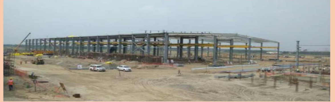
CONSTRUCTION IN FULL SWING AT MADHEPURA
