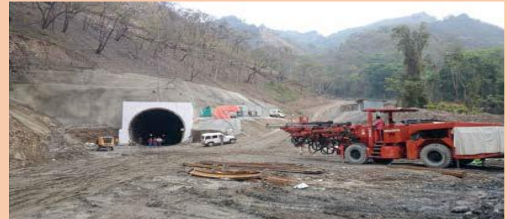
LONGEST RAIL TUNNEL COMPLETED IN NORTH EAST
